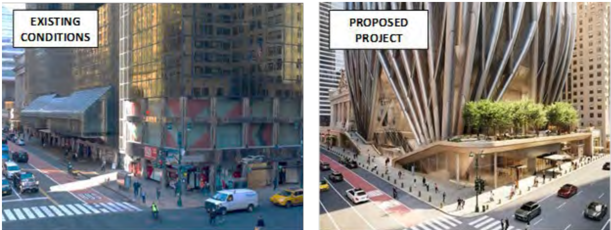
View facing northwest of the southern corner of 175 Park Avenue at the intersection of East 42nd Street and Lexington Avenue Source: Renderings by Skidmore, Owings & Merrill, 2021.
