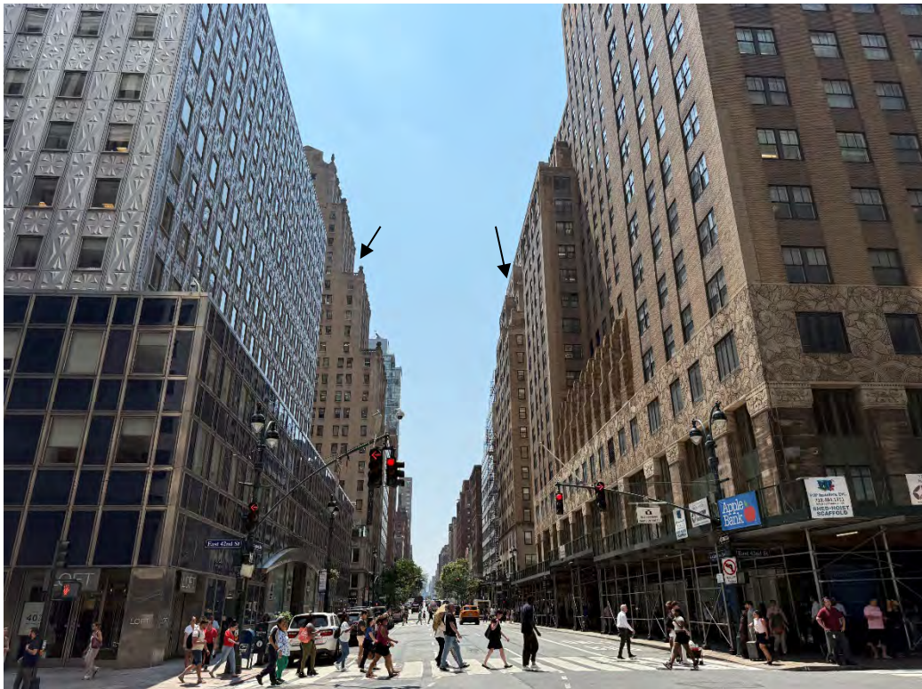
10. Map ID 16: 364 Lexington Avenue (right arrow) and Map ID 15: 363 Lexington Avenue (left arrow) in Lexington Avenue context. Chanin Building and Socony-Mobil Building in foreground (right and left, respectively). Photographer facing SW.
