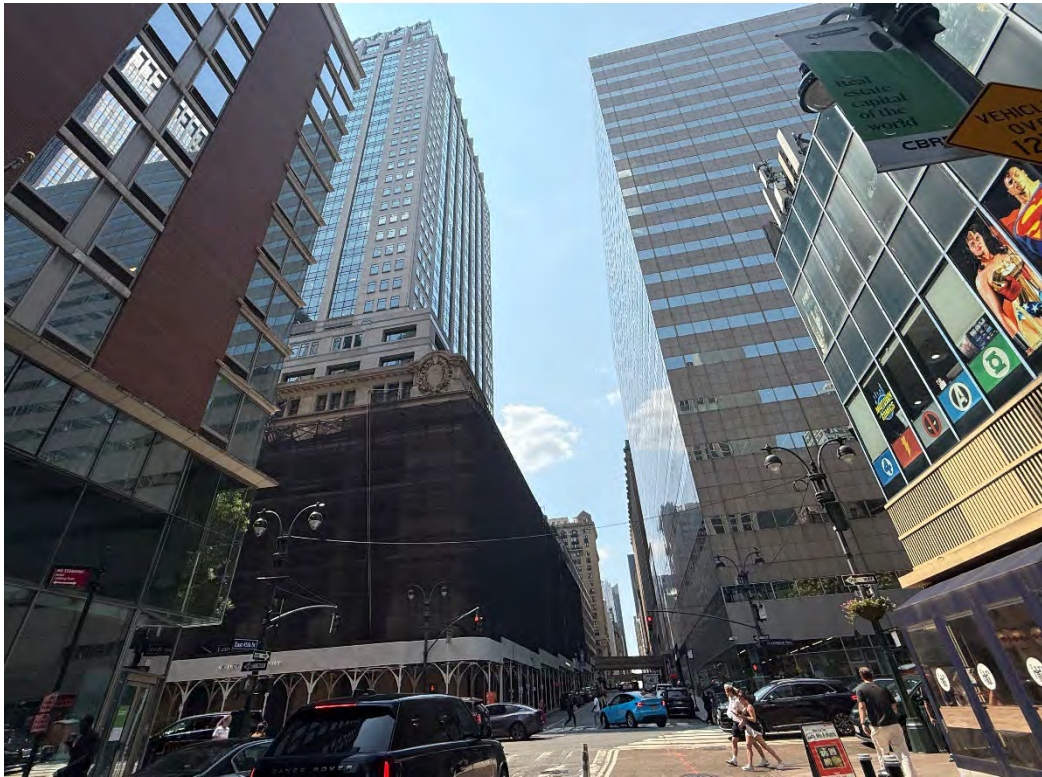
28. Map ID 4: Grand Central Terminal Post Office (under scaffolding), 450 Lexington Avenue, and East 45 th Streetscape. Photographer facing W.
