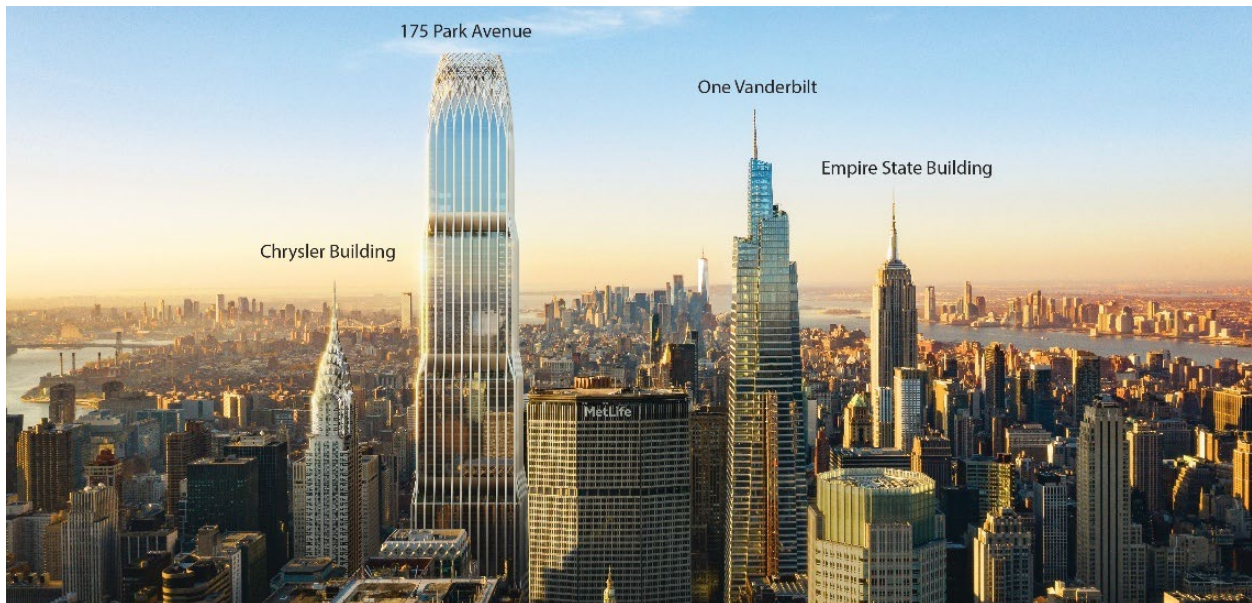
Rendered view facing southwest showing 175 Park Avenue amidst the East Midtown skyline in the Proposed Action.
